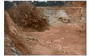
Figure 1. Flyrock at bench blasting
